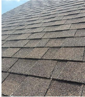
Significant granule loss around edges of shingles
